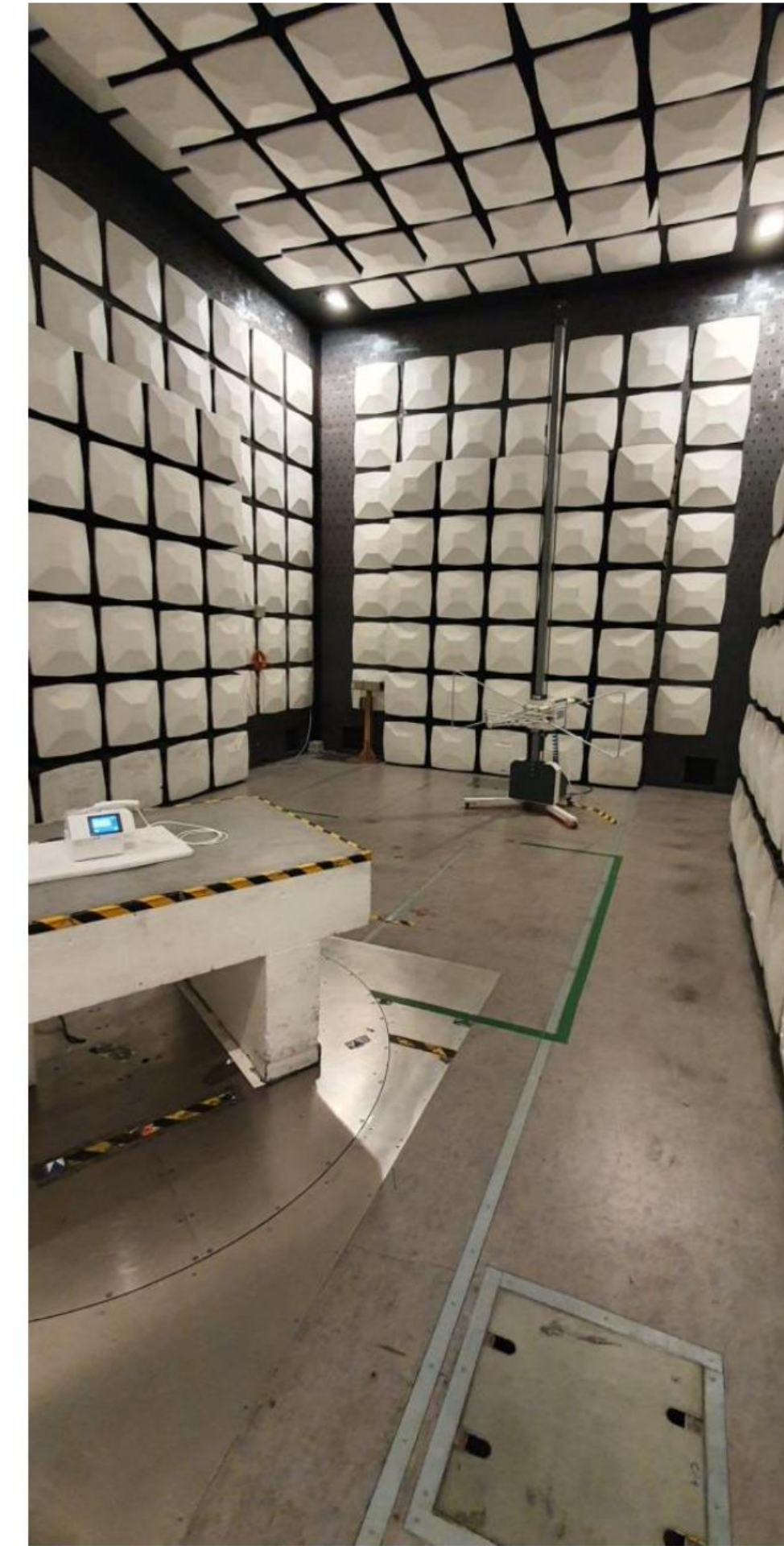
RF chamber at ELEMASTER
